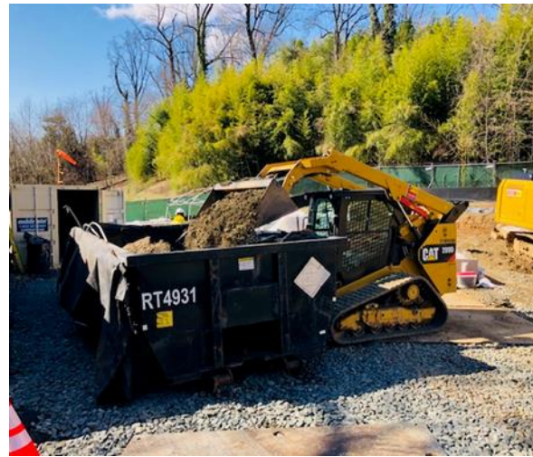
Loading Soil in Roll-Off
