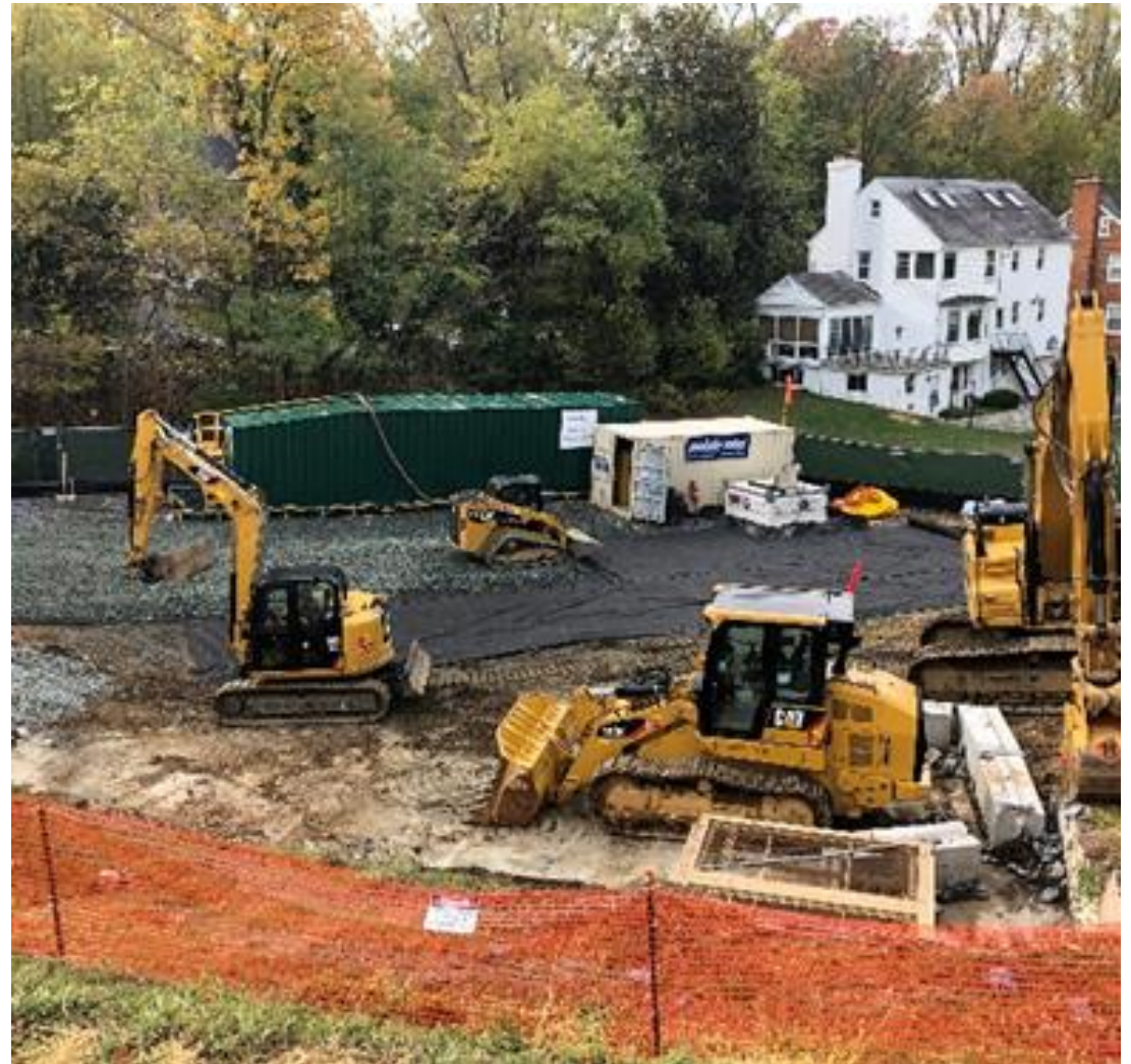
Overview of Previous Remediation Operations
