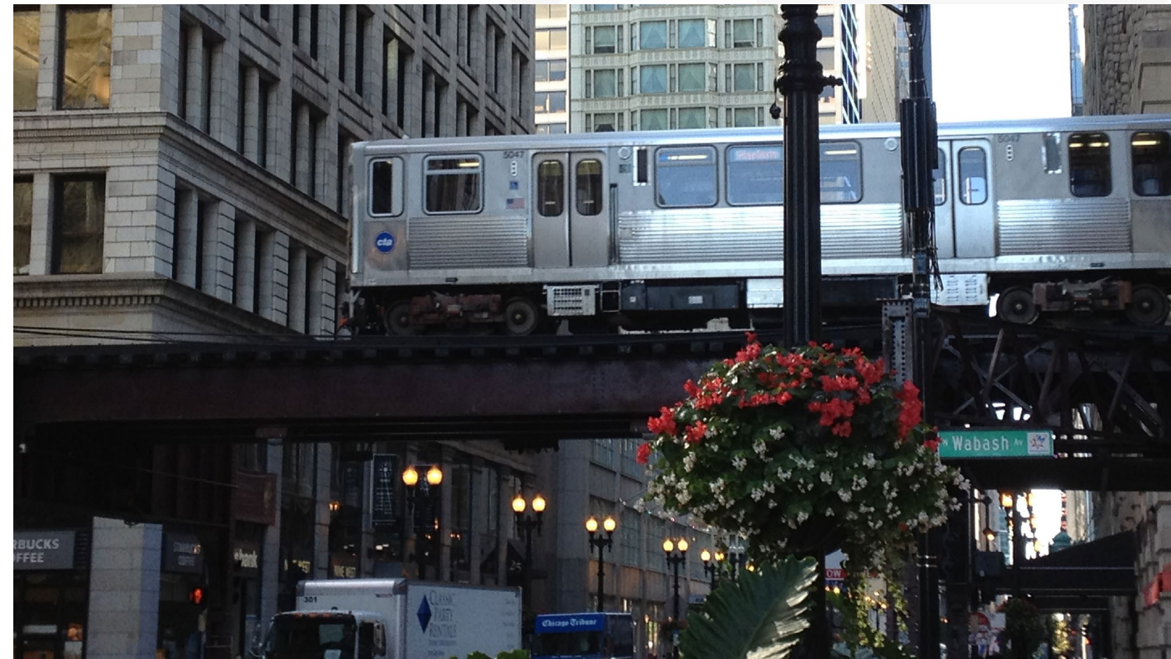
Elevated train in Chicago
