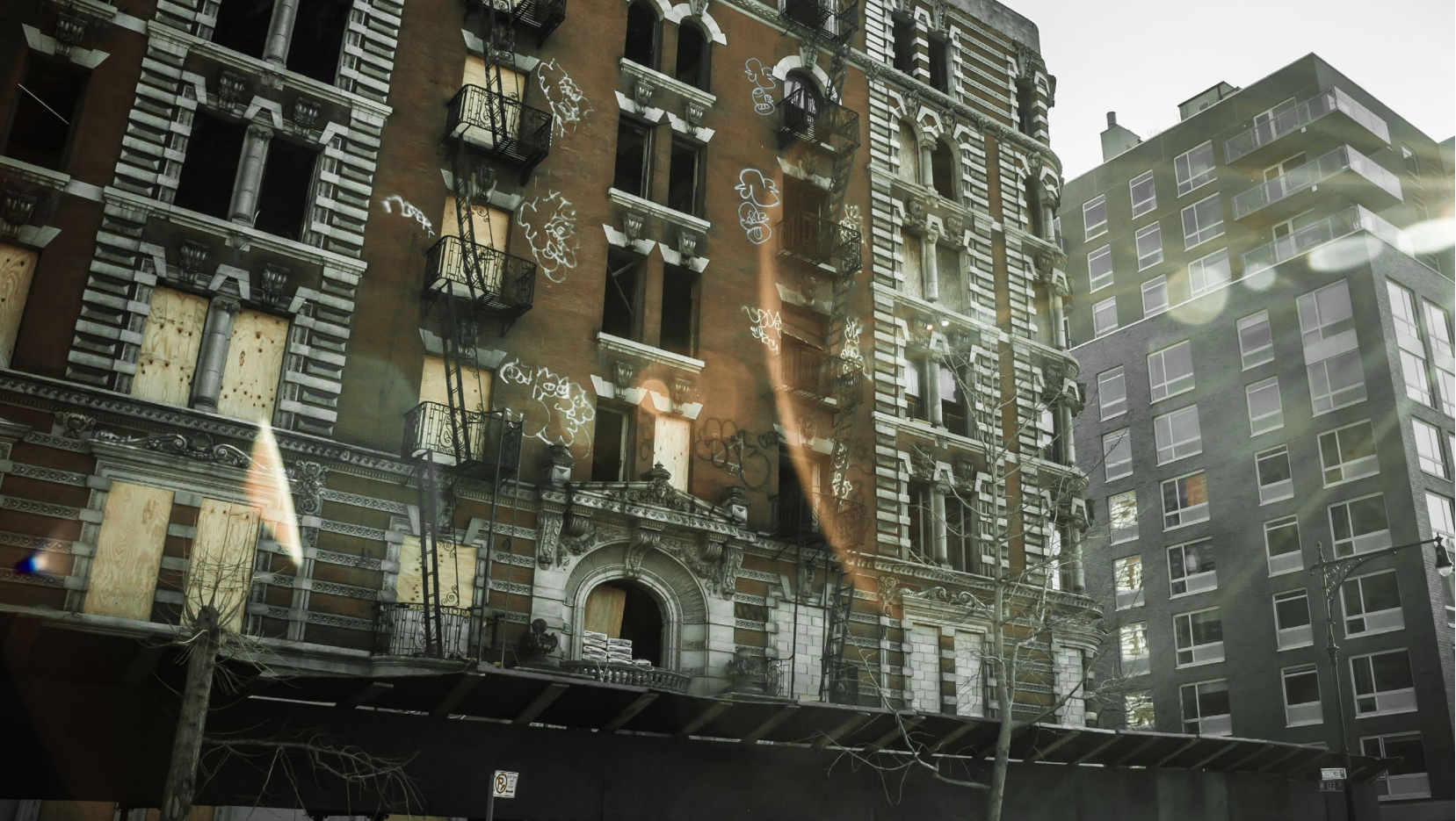
Decaying buildings in Harlem
